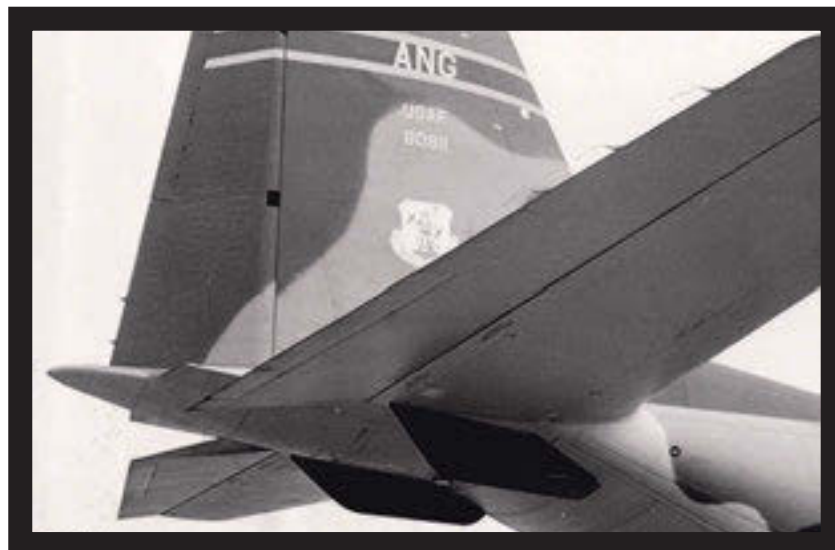
Twin fins jut down from the horizontal stabilizer of a C-130E. Although the fins were added to improve fuel consumption in the early 1980s models of the Hercules, they didn't improve the plane's speed of 335 MPH. (Lockheed photo)
